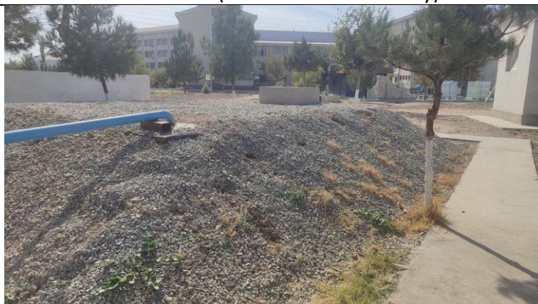
In Ground Water Tank (Karshi State University)
